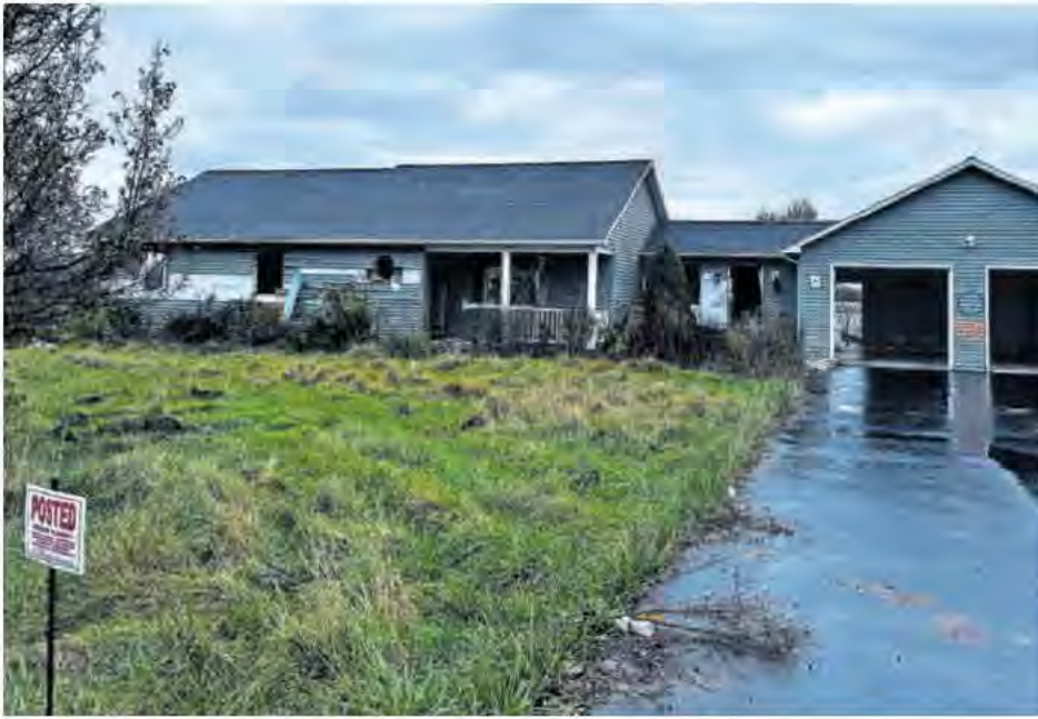
This home is one of about 12 that remained standing on Burnet Road in Clay as of Nov. 9. Glenn Coln, gcoln@syracuse.com
