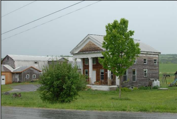
Figure 32. 4843 Old Country Road, Town of Smithfield. Representative nineteenth-century farmstead with a Greek Revival residence within the Historic Resources Study Area.
