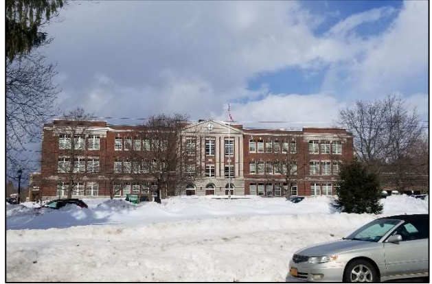
Figure 27. Cazenovia Central School (USN 05344.000344), Village of Cazenovia. Representative public-school building within the Historic Resources Study Area.
