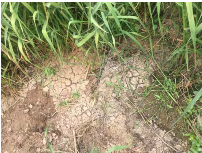
Mud cracks, change in vegetation type and density.
