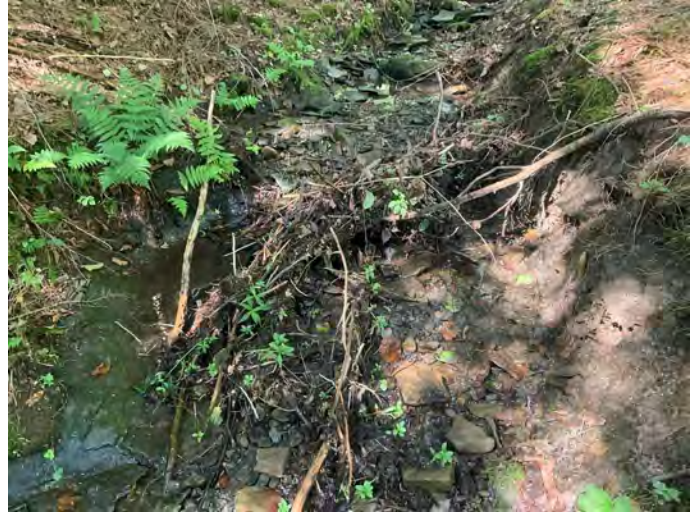
Wracking, break in slope, change in particle size distribution
