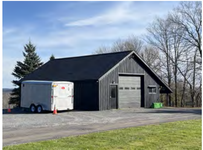
Dorothy Riester House and Studio (aka Hilltop), shed, facing southeast
