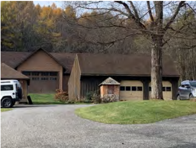
Nichols House, outbuildings, looking west
