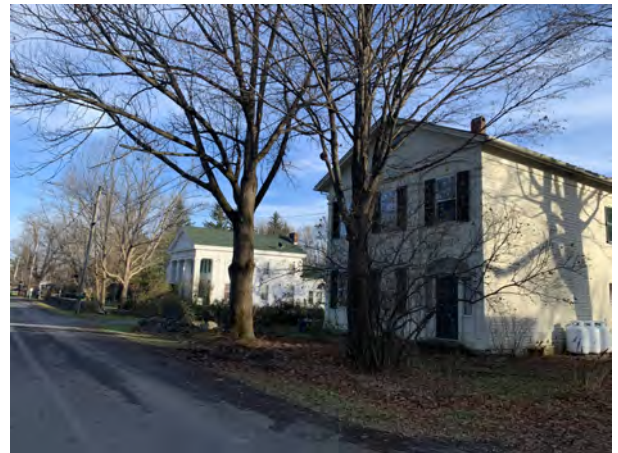
4694 and 4690 Park Street, view southeast
