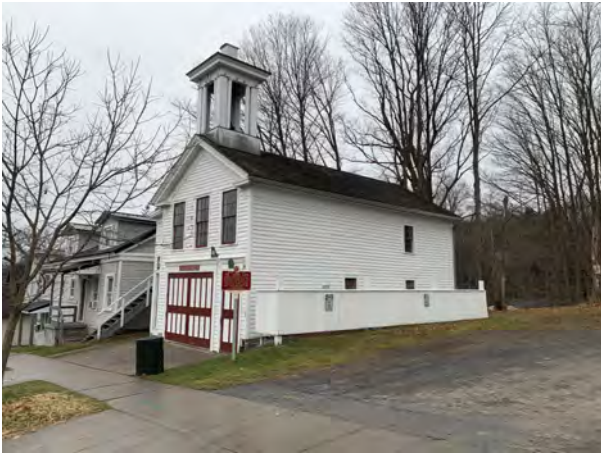
Morrisville Engine House
