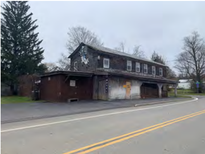
North and west elevations
