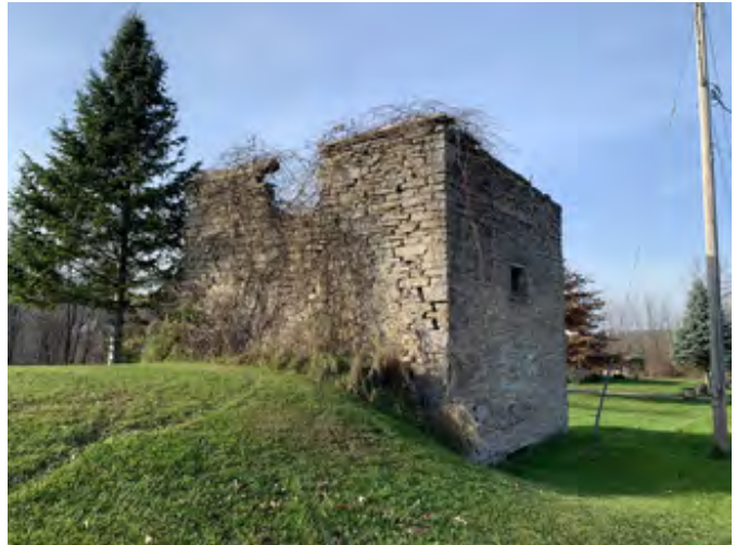
South and east elevations
