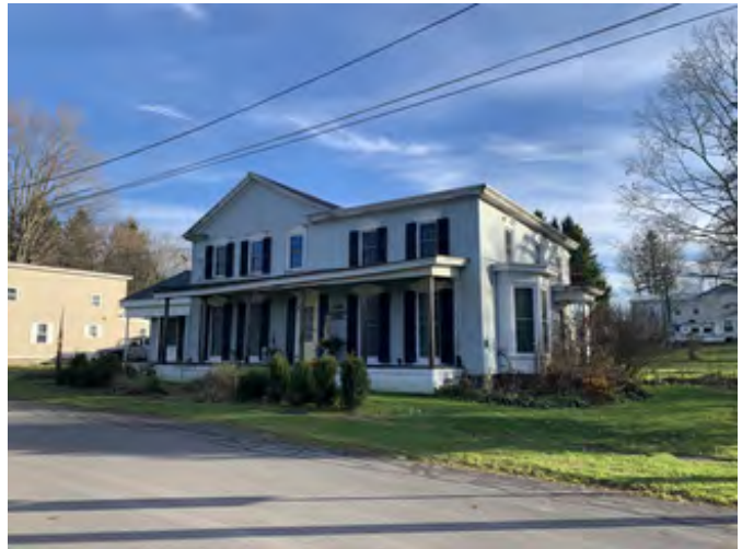
North and west elevations
