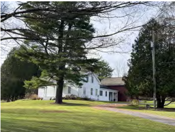
Case House, facing southwest
