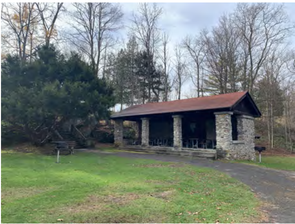
Picnic shelter, view northwest
