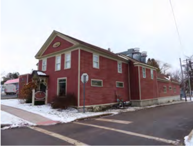
North and west elevations
