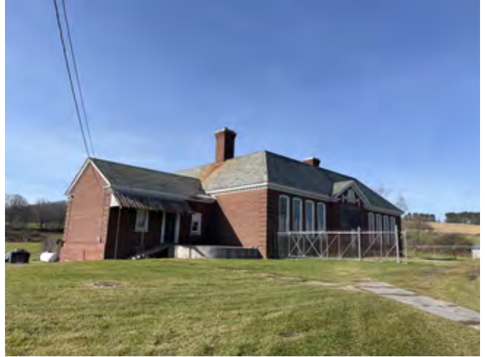
Eaton Grade School, looking northwest
