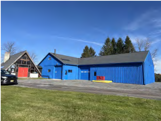
Dorothy Riester House and Studio (aka Hilltop), visitors center and barn, facing northeast
