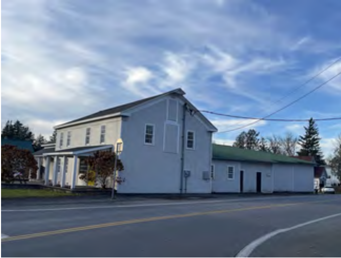
South and east elevations
