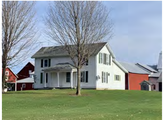
Residence, west and south elevations
