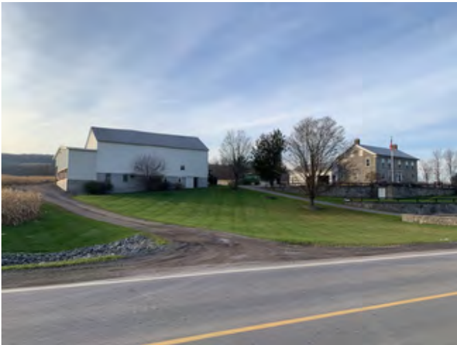
Barn and residence facing northwest
