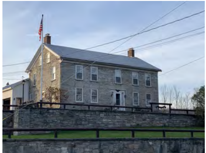
South and east elevations
