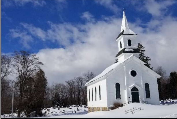
Figure 26. Nelson Welsh Congregational Church (93NR00504), Town of Nelson. Representative civic/religious building within the Historic Resources Study Area.
