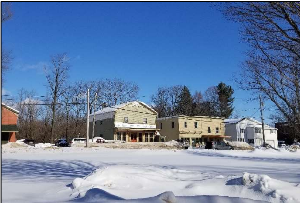
Figure 28. Italianate-style and vernacular commercial buildings, hamlet of Peterboro. Representative nineteenth-century commercial buildings within the Historic Resources Study Area.
