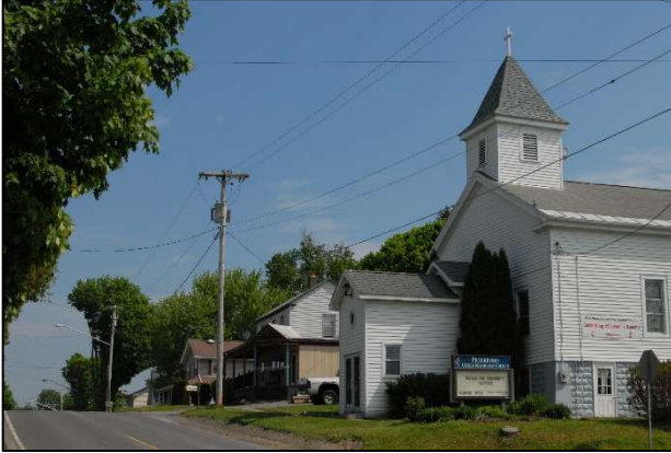
Figure 20. Peterboro United Methodist Church, 5240 Pleasant Valley Road, hamlet of Peterboro, Town of Smithfield.
