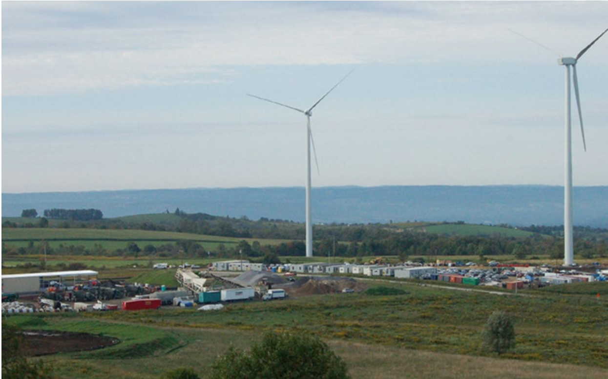
Figure 5.2-5. Construction Staging and Laydown Area
