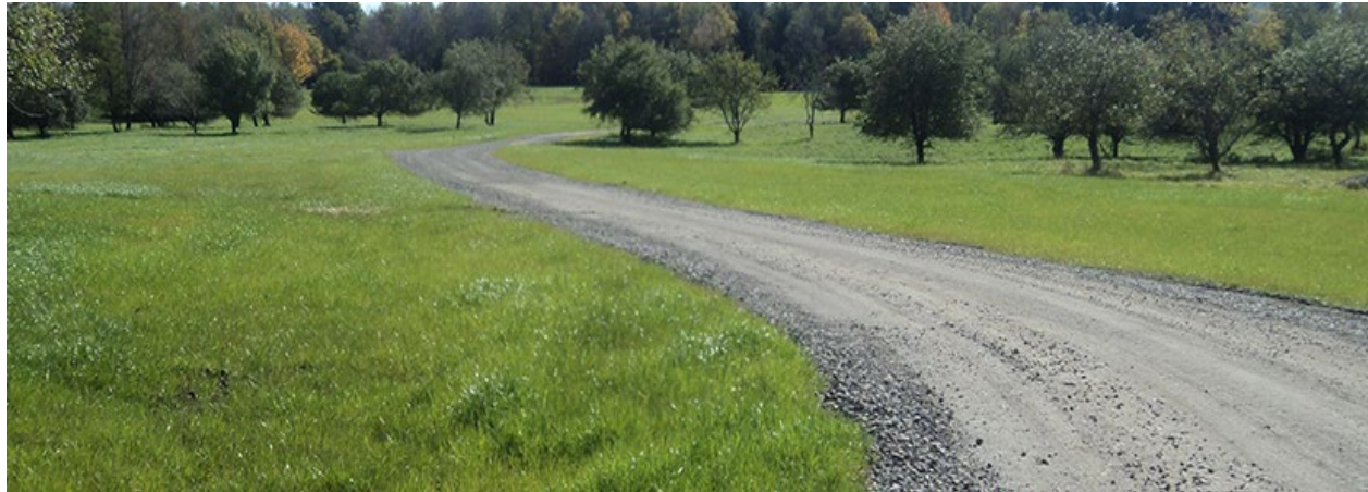
Figure 2.2-7. Representative Photo of a Turbine Access Road
