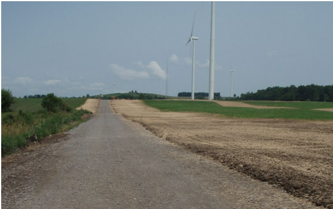
Figure 5.2-9. Stabilization and Restoration of Temporarily Disturbed Soils
